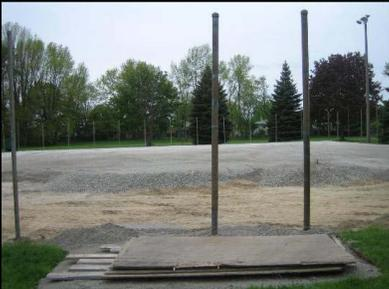
Phase 1 began with site surveys, prep work to mark around electrical and the 30 year old fence being removed by the City of Mississauga. Equipment was brought on site to excavate and remove the two existing courts and layers of penetration material. Granular A was brought on site to fill the courts and 2" of HL3 surface course asphalt was applied. You will note that there is an extra box area paved which will host the port-a-let bathroom and equipment box.
